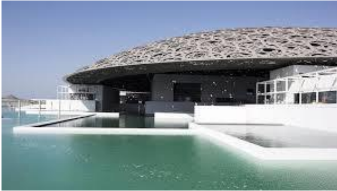
Figure 4 The Louvre Abu Dhabi - F# was used for the digital 3D model to manufacture the roof
